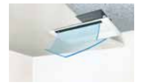
(1) One-direction "down-blow" system
